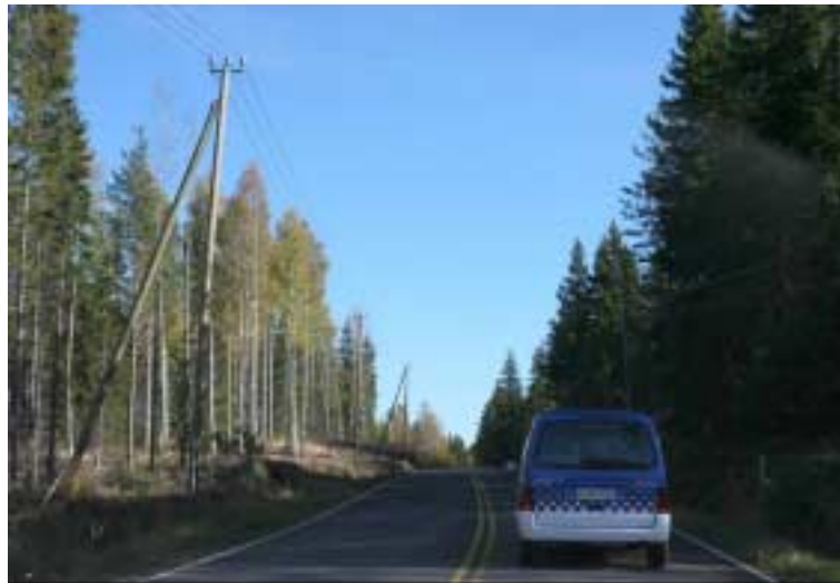
Figure 5.5. Covered conductor PAS overhead line along the roadside.
