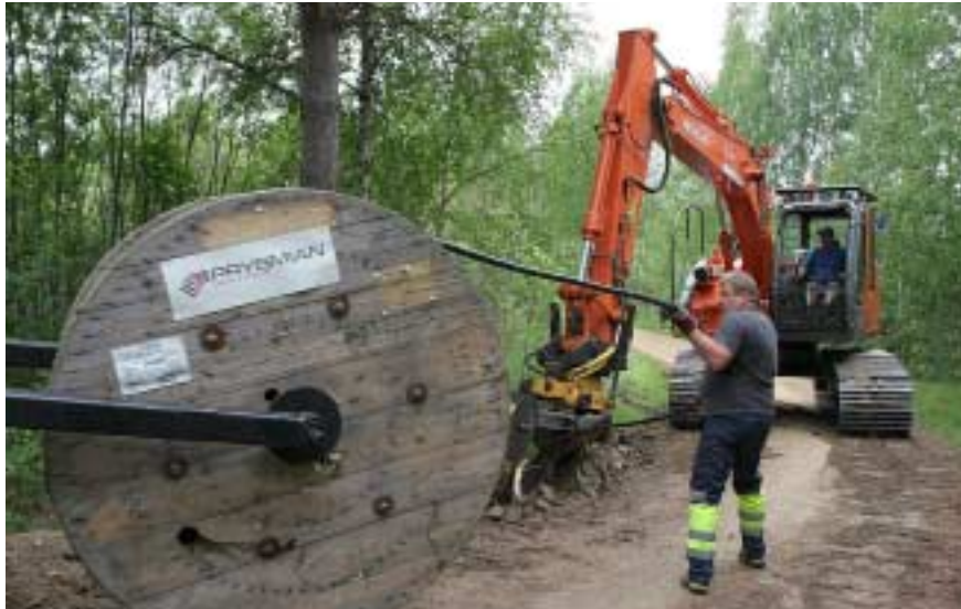
Figure 5.4. Ploughing of a low-voltage underground cable.
