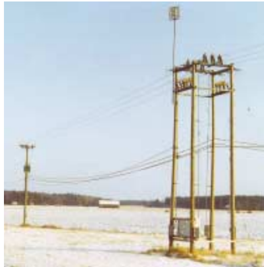
Figure 5.11. Remote-controlled disconnector substation.
